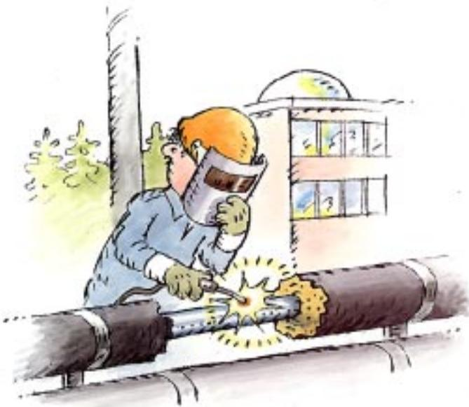
*In order to avoid poisonous gases, the layer of paint and isolating foam should be completely removed by at least 25 cm on each side of the welding place.*
